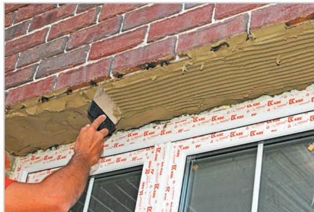
2. Apply the adhesive mixture to the supporting surface of the building. When applying the mixture the grooves from the filling knives should be along the processed surface.
