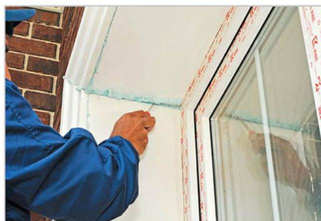
12. After thorough drying, cut down the excesses of the dried fixfoam. If cavities are detected, re-coat with fixfoam, wait until the surface is completely dry, and if required, cut down the excesses once more.
