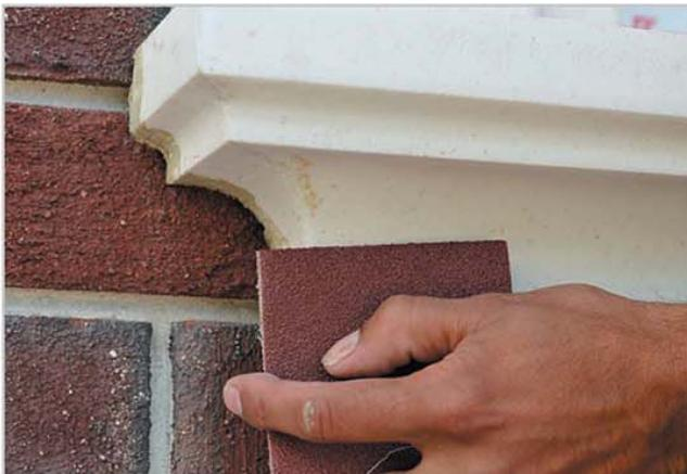
17. After thorough drying of the DarMix decorative and restoration mixture, smooth the joints and the renovated places with sand paper.
