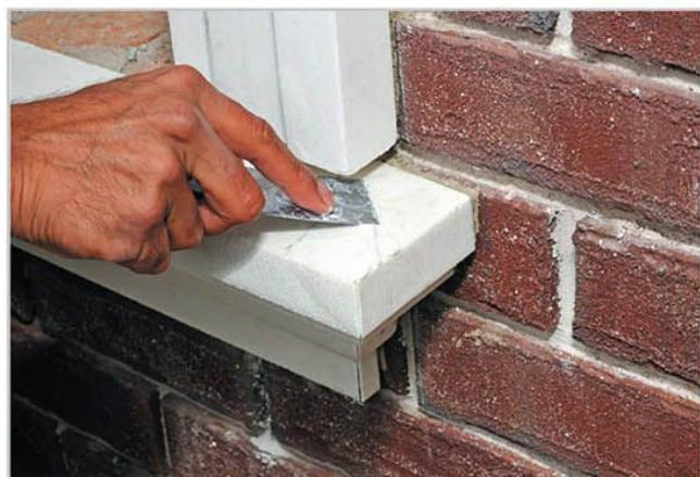
16. Cover the ready joint places with the DarMix decorative and restoration mixture using a filling knife, densely pushing the mixture into the weld.
