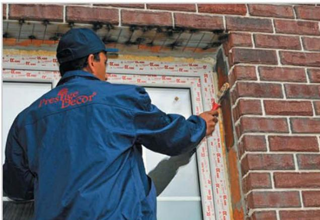
1. Remove any cement mortar, salt efflorescence, mould, dust and other pollutions from the supporting surface. Apply facade primer.
